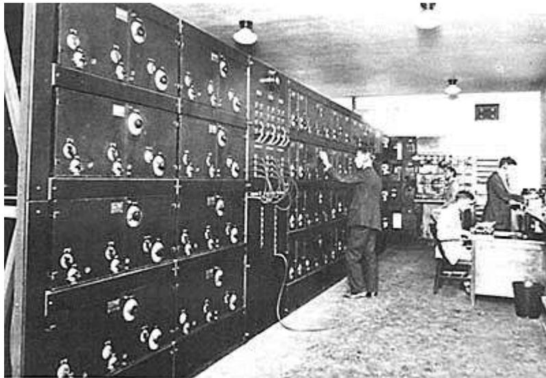
Figure 4. Rows of Receivers at the Belfast, ME Station
