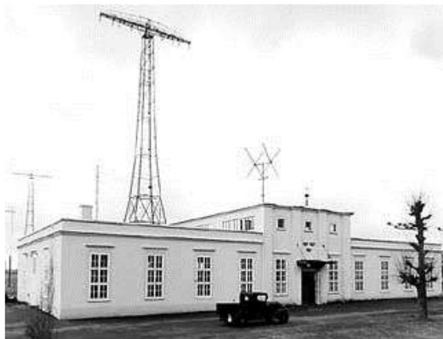
The transmitter building at Grimeton. Two of the six 127-meter antenna masts are visible.
